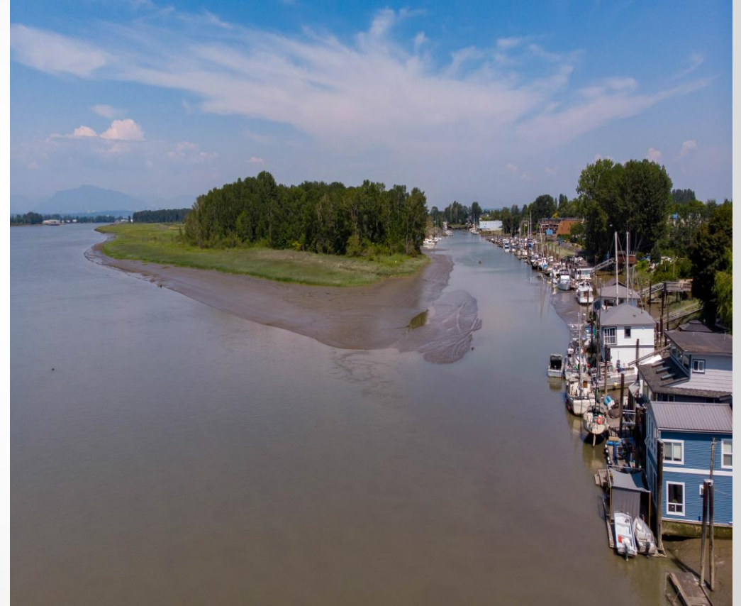
Ladner Harbour Entrance
